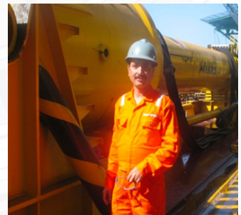
Attending Installation of Pile Foundation for Offshore Platform
