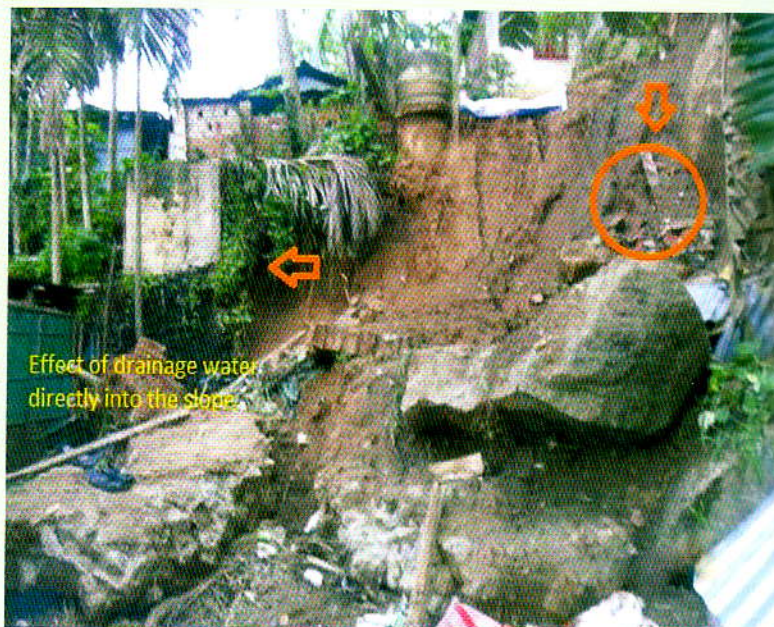
Fig-2: Landslide Caused due to Water Falling in Slope in Absence of Proper Drainage System (Shantipur Hill Side)
